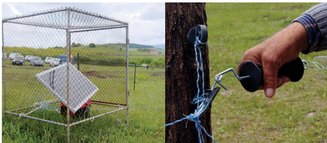
Pic. 27. Installing electric fencing on the pilot pasture of Ganakhleba village
